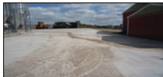
Completed concrete pad for silage leachate system.
