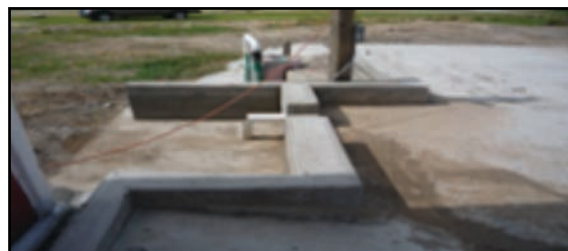
Completed silage leachate collection system.
