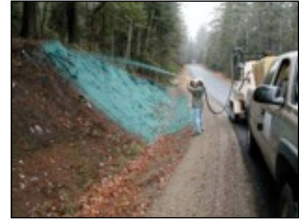
Road ditch hydroseeding
