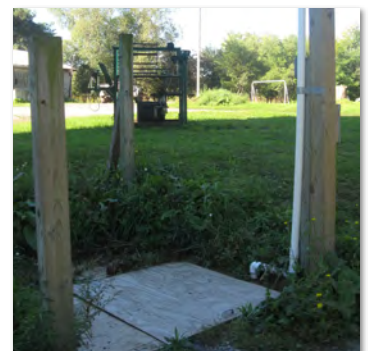
Milkhouse Waste Collection System
