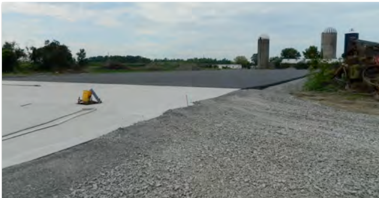
Bunk and concrete apron
