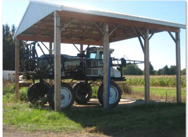
Covered Agrichemical Mixing Facility
