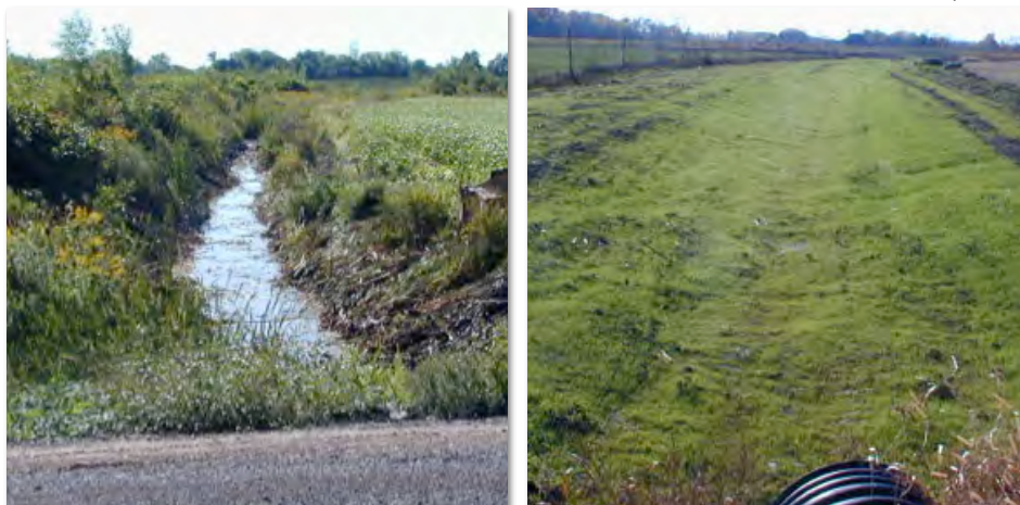
Example of grassed waterway, before and after.
