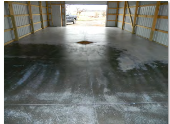
Ag chemical handling facility
