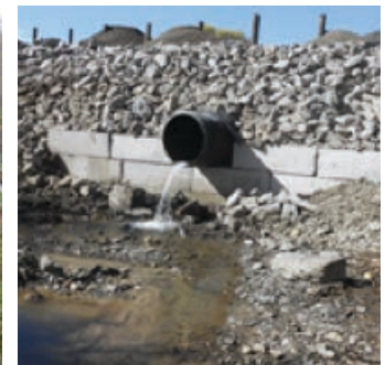
A cross culvert was extended 20 feet on Scipio - Booth Road in the Town of Scipio.
