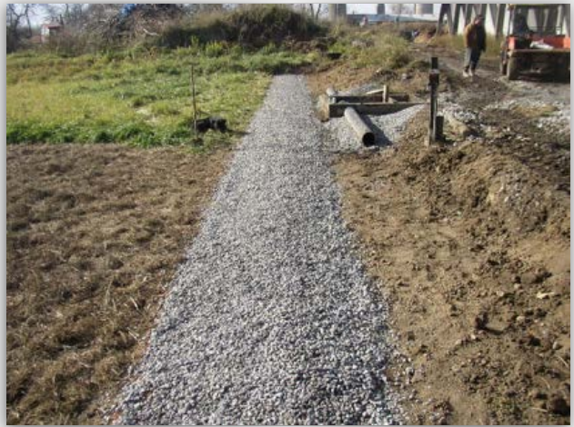
Silage leachate collection system. Photo credit: Niagara County SWCD
