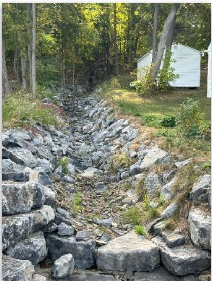
Stormwater runoff from State Route 54 has caused severe gully erosion along East Lake Road which resulted in over 250 cubic yards of material entering Keuka Lake, a AA drinking water resource for residents of Steuben County.
