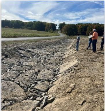
The road ditch on Welker Road in the Big Stream Subwatershed of Seneca Lake had been subject of erosion for many years despite efforts to stabilize the flow. Over 150 linear feet of rock paving was determined to be the best solution to protect the bed and banks; while allowing the velocity to remain high at the county box culvert.
